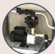
Pump pre-installed with rain/mains changeover
